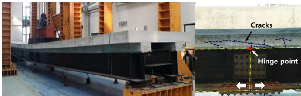
Fig. 10 Failure and crack pattern of concrete at bolted connection of girder
