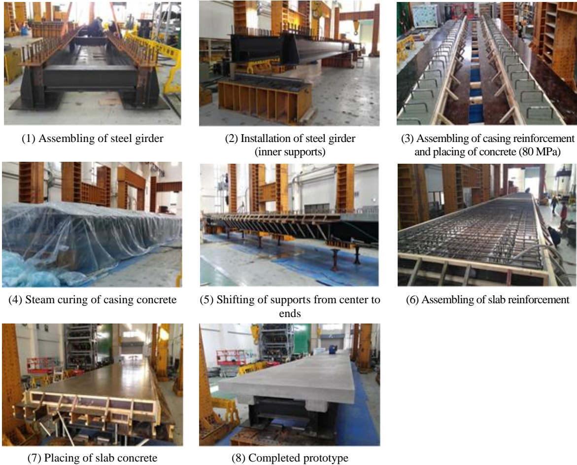
Fig. 4 Sequential fabrication of hybrid girder prototype
