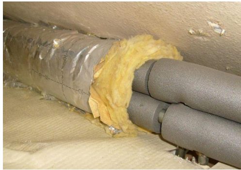
Fig. 1.3 Mineral wool wire pipe thermal insulation.
