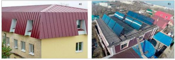
Figure 3 Examples of increasing the stability of the living environment of an object: a) a superstructure of a building using the attic, b) placement of solar elements on the roof of a building
