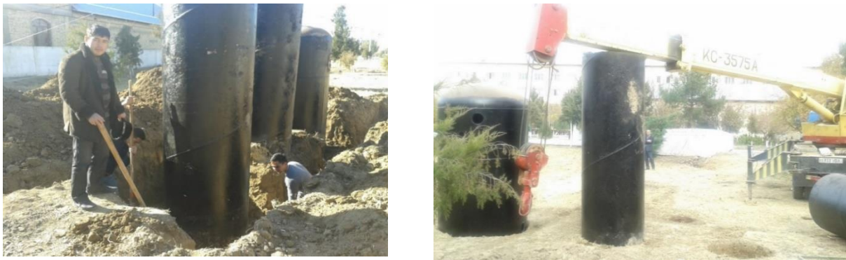
Figure 1. The process of building a lysimetric complex on the territory of the Karshi Engineering-Economics Institute.
